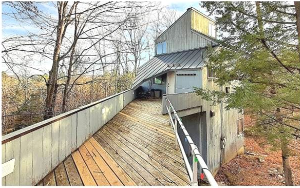
106 Upper Loop | Ludlow Located in the desirable West Village area, this home offers deeded ski access to Okemo's Sachem Trail website link: https://bit.ly/3X5pu1D
